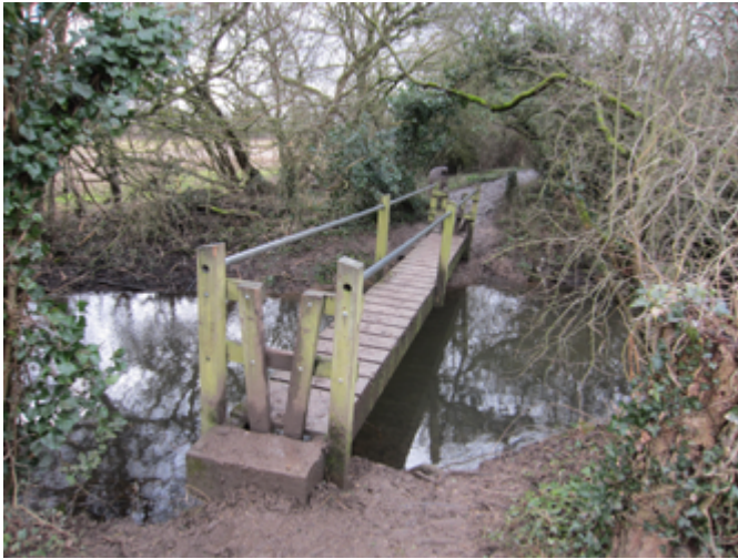
Bridge before improvements
