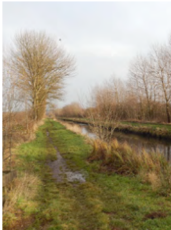
Bottesford Beck before P4C improvements
